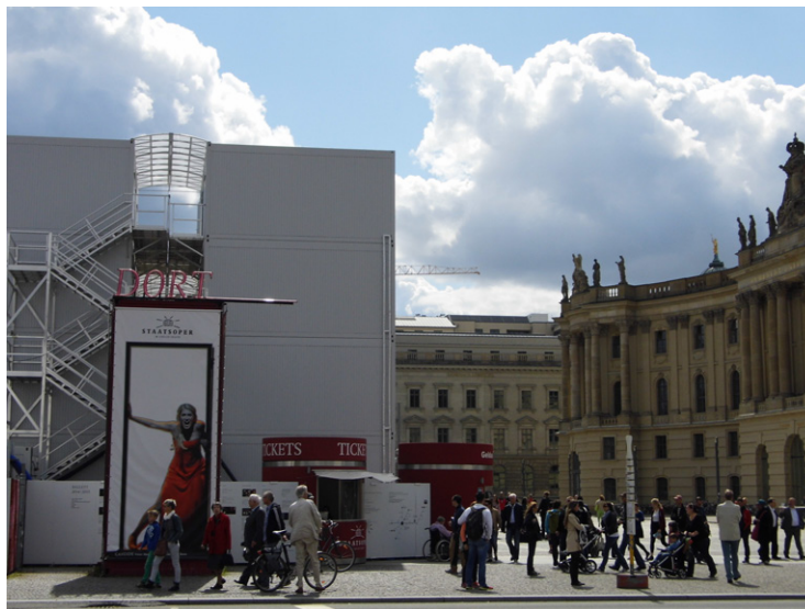
Figure 5: Bebelplatz with construction containers
